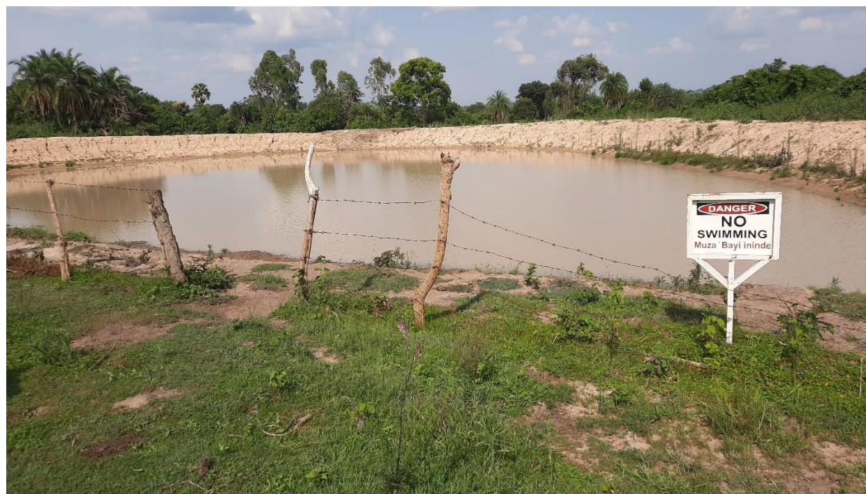
Figure 6 One of the infrastructure projects (water ponds) constructed
