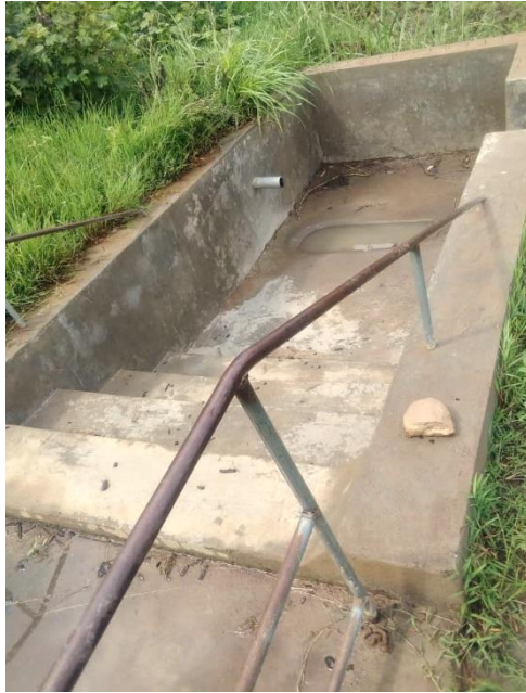
Figure 9 Spring protection infrastructure project
